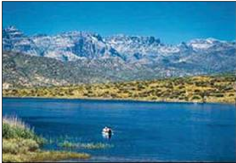
Figure 2.11 Photograph of Clanwilliam Dam
